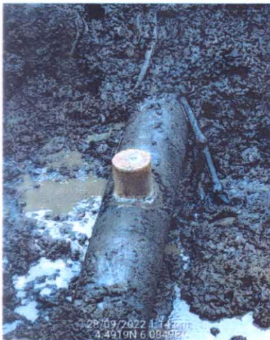
FIG 2-3: Incident Facility repaired and Aqua wrapped
